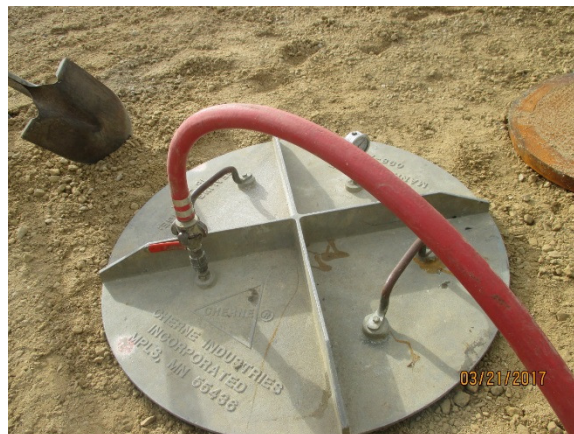
Vacuum testing a precast gravity sewer manhole
