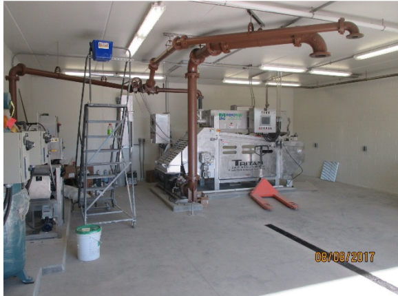
Overall view of the completed Sludge Press Room.
