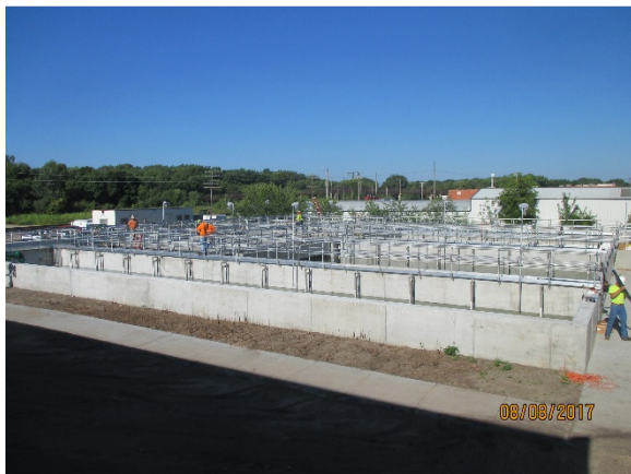
Overall view of the completed Aero-Mod tank
