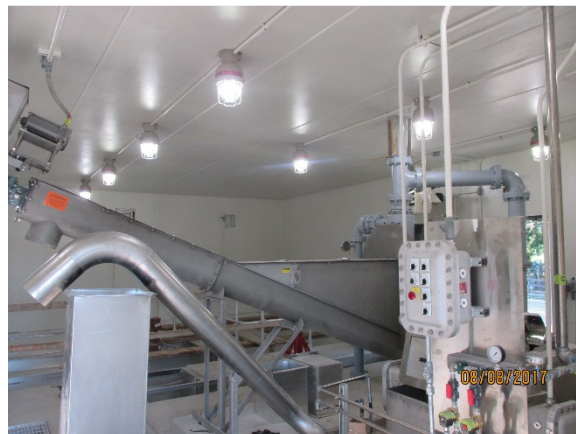
Overall view of the completed Headwork's Room
